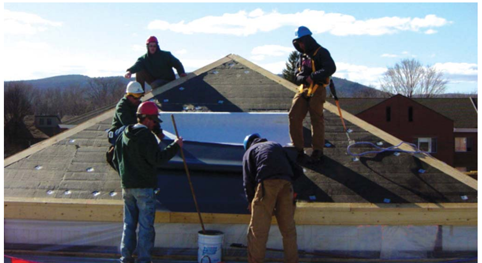
Workers install Sarnafil's Décor Roof System on one of the pyramids.
